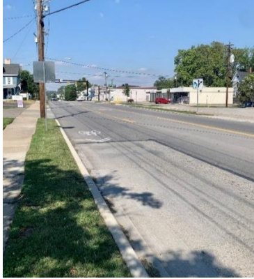
Image 5: North Pike Existing Streetscape
